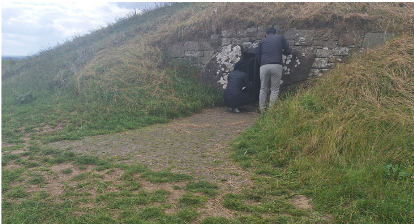
Plastic grid ground reinforcement seldom establishes vegetation and can detract from the ambience of naturalistic or historic sites. Photo : Mitchell + associates
